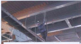
Most of the work will be executed by blast and paint crews inside tented containment areas. The containment areas are erected by enclosing the sides of the bridge completely with canvas curtains.
